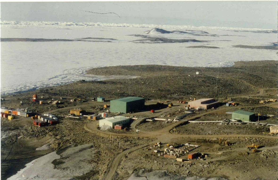
Operations building, foreground right.
